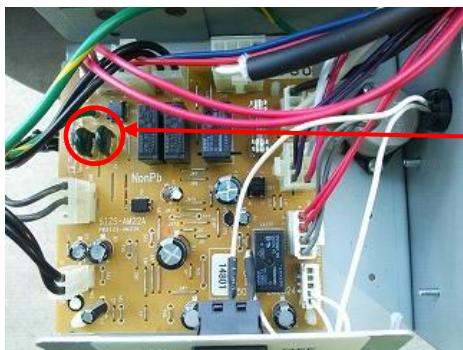
Picture 9 Inspection surge absorber (SA)
